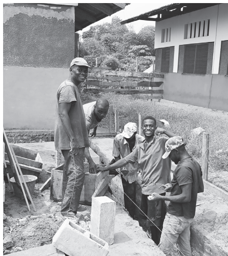
Construction on the building projects at the Vanga Evangelical Hospital.
